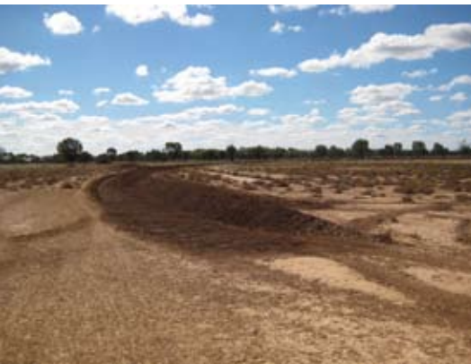
Banks are used for 'water ponding' – to change the way water moves across the landscape, reducing sodic scalds and erosion.
